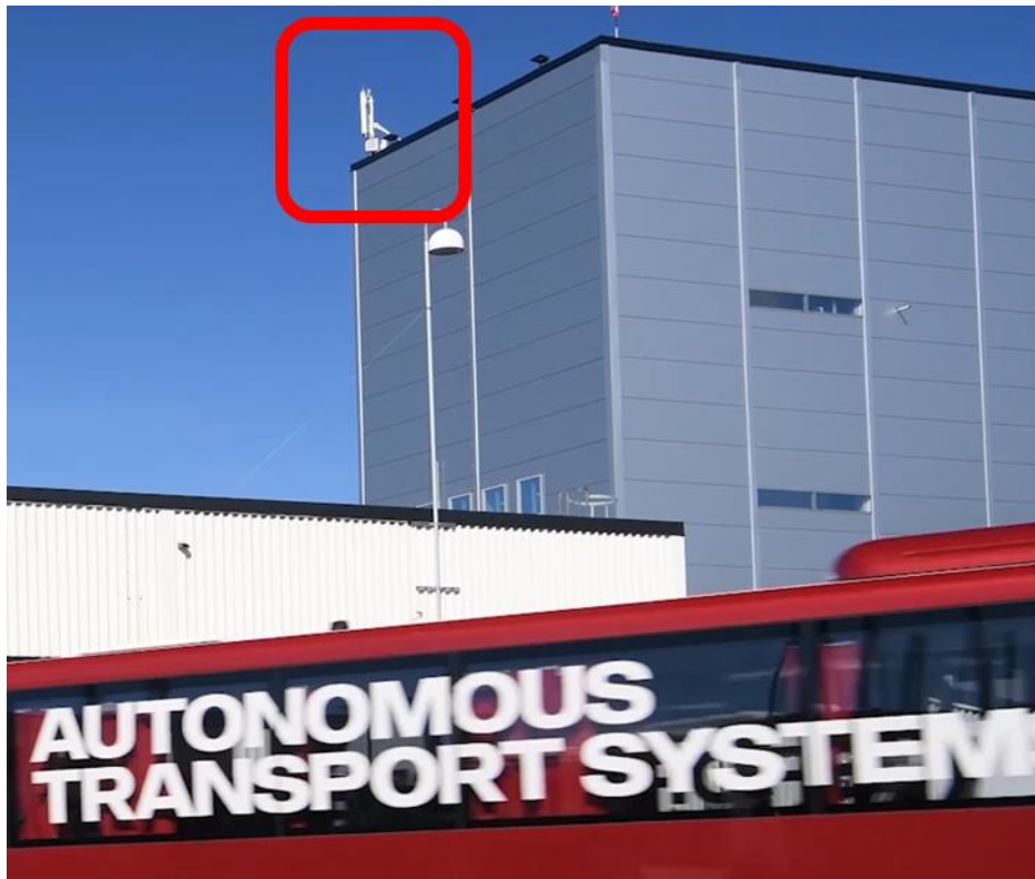
Figure 56 – Proof Of Concept 5G antenna pictured on top of the Scania wind tunnel above iQPilot vehicle #1 (zoomed in from Figure 6)
